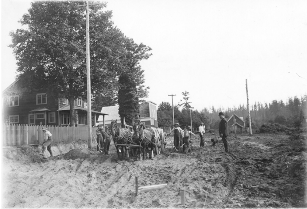
3d St. being graded D.C.Campbell house * V.J.Kelly barn - Everton house & barn
